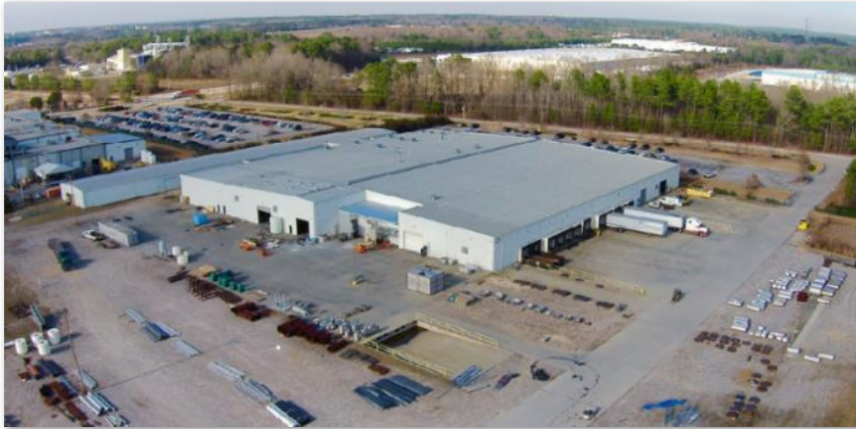
AVANTech Facility – Columbia, SC
