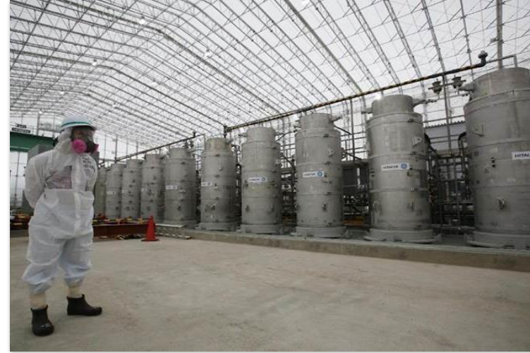
HERO (Gen-2) Fukushima – 2015 Used Cooling Core to Increase Ci Loading
