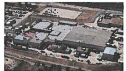
Plutonium Facility 4 at Los Alamos National Laboratory
