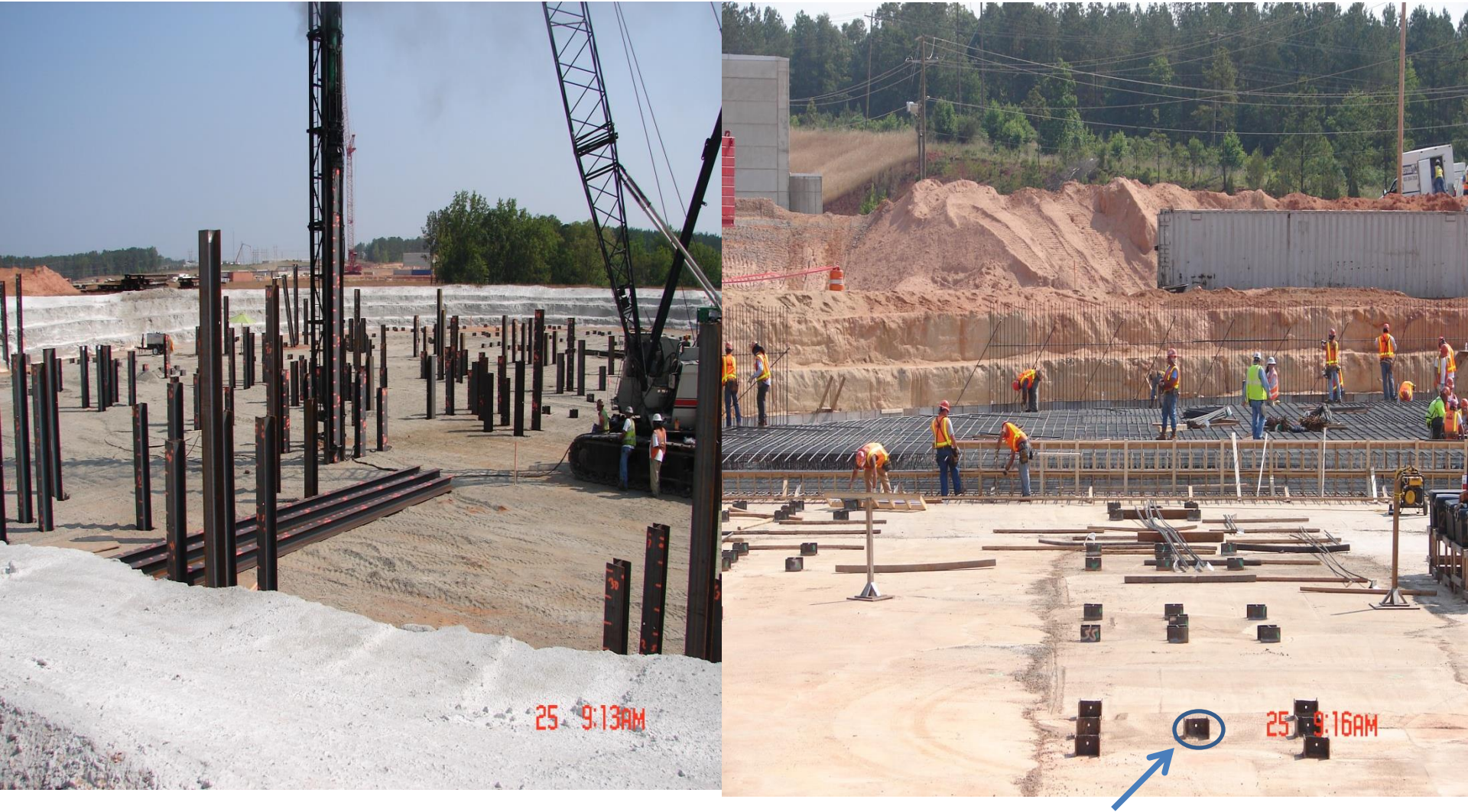
Rebar is "tied" to piles
