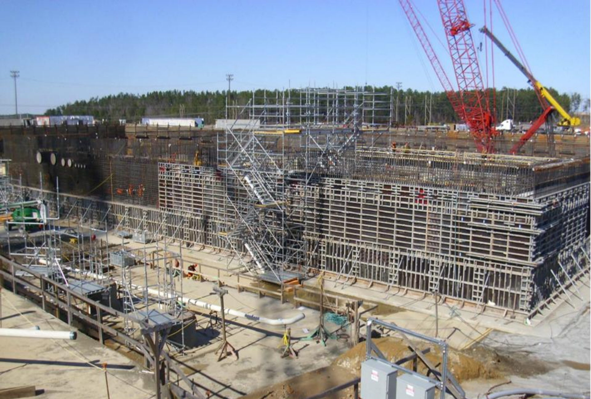
Unit 2 Turbine Island 1/31/2013
