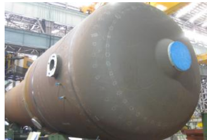
Upper internal welding of Final Vessel for Unit 2B SG
