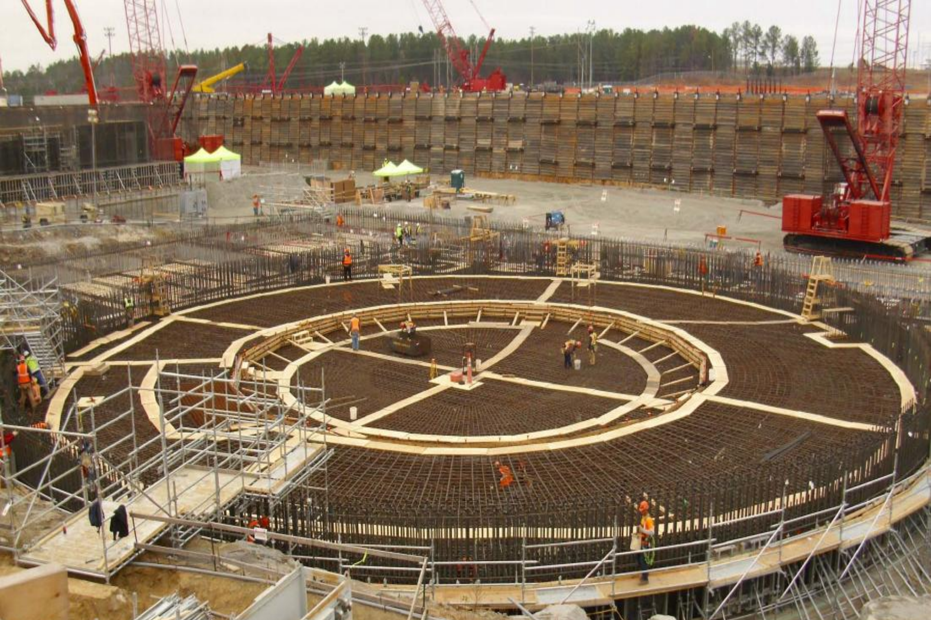
Unit 2 NI Shield Building 12/7/12
