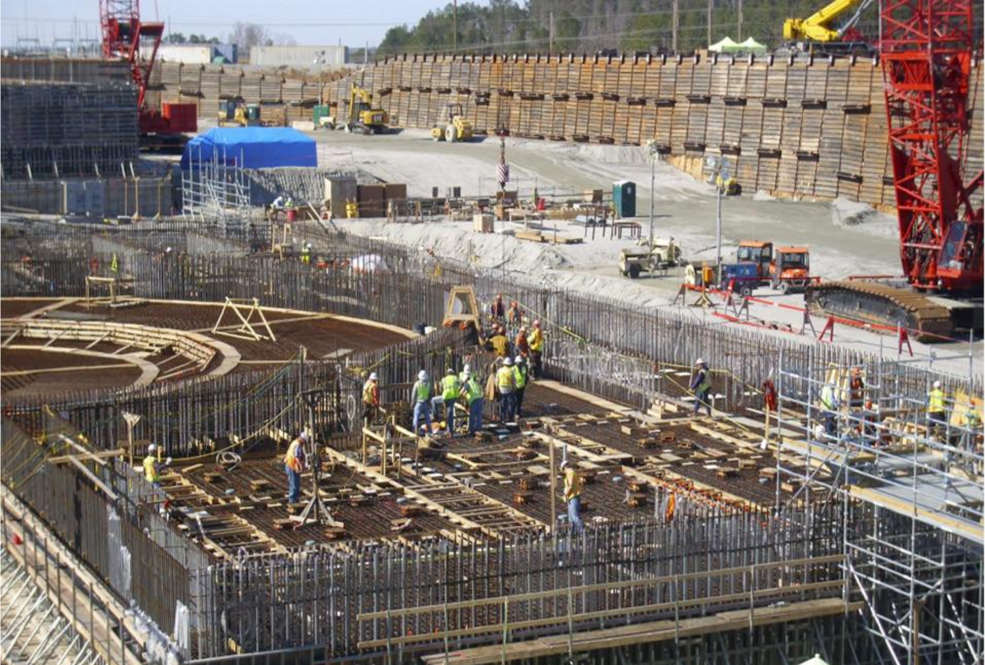
Unit 2 NI Basemat South End 2/9/2013
