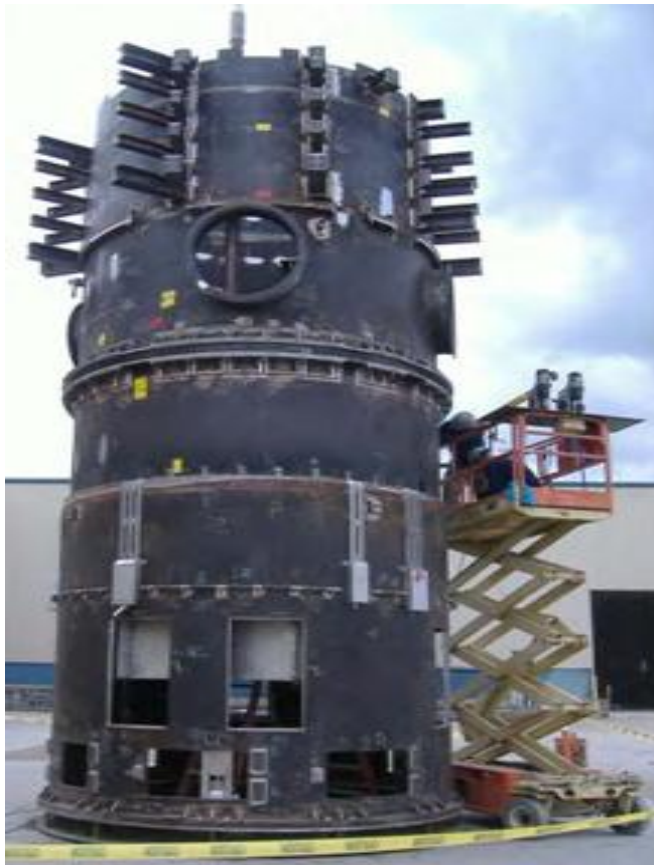
U2 Integrated Head Package Fit-up
