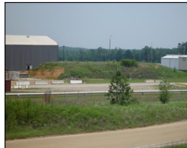
June 2005 Soil Covering
