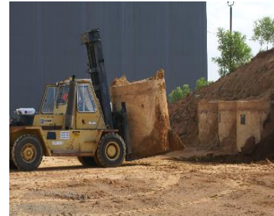
June 2009 Begin Culvert Retrieval
