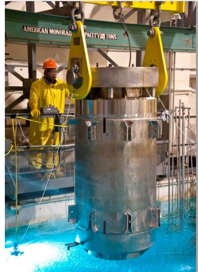
Spent Fuel storage in L Basin
