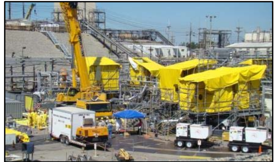
Tank 12 Tank Top Preparations
