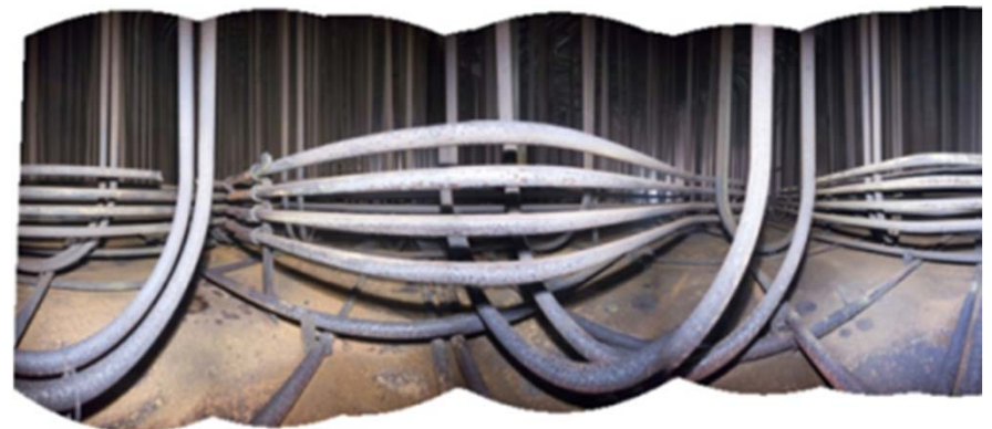
Tank 12 Post-Chemical Cleaning
