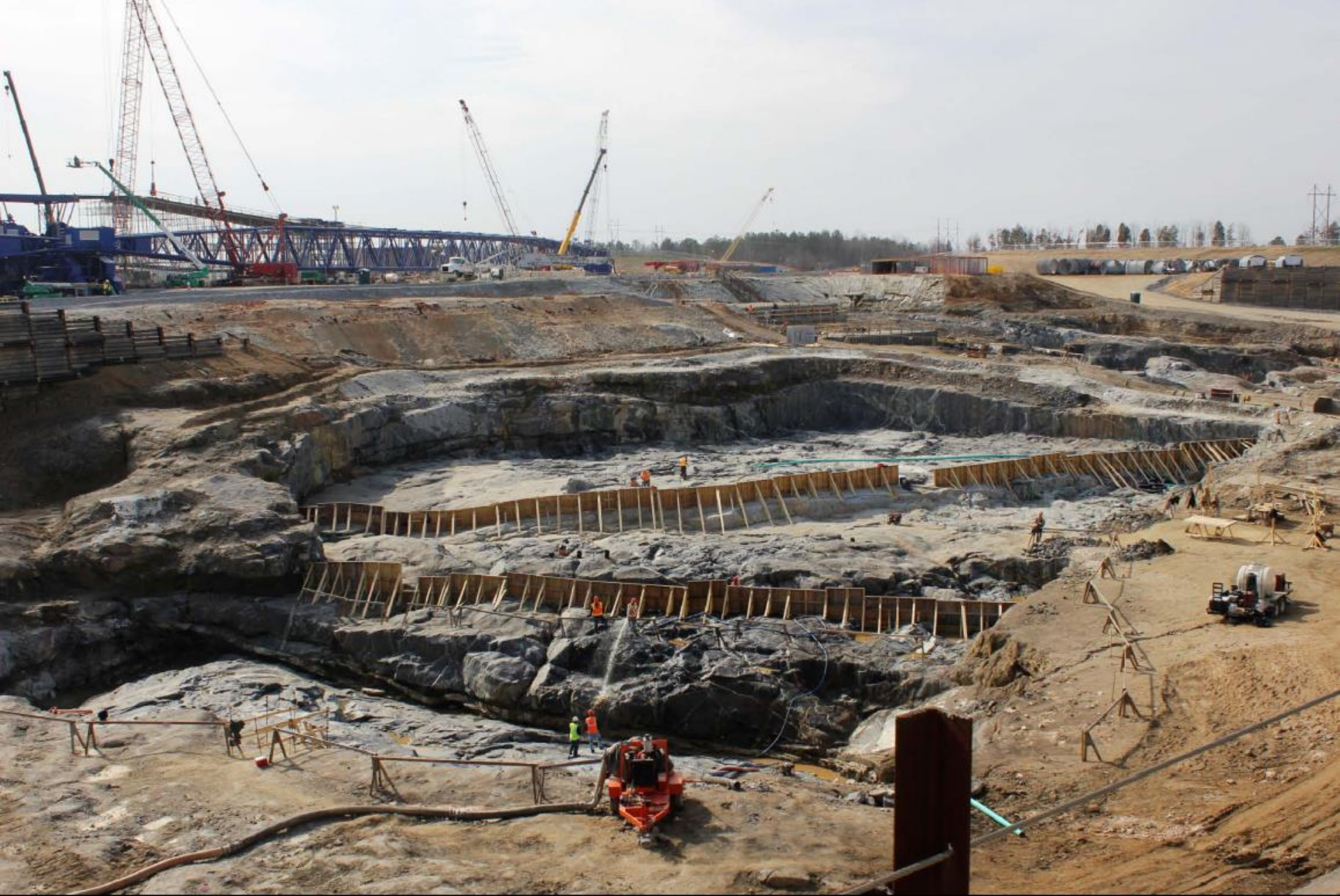
02. 09.12 Unit 2 Formwork and Rock Cleaning
