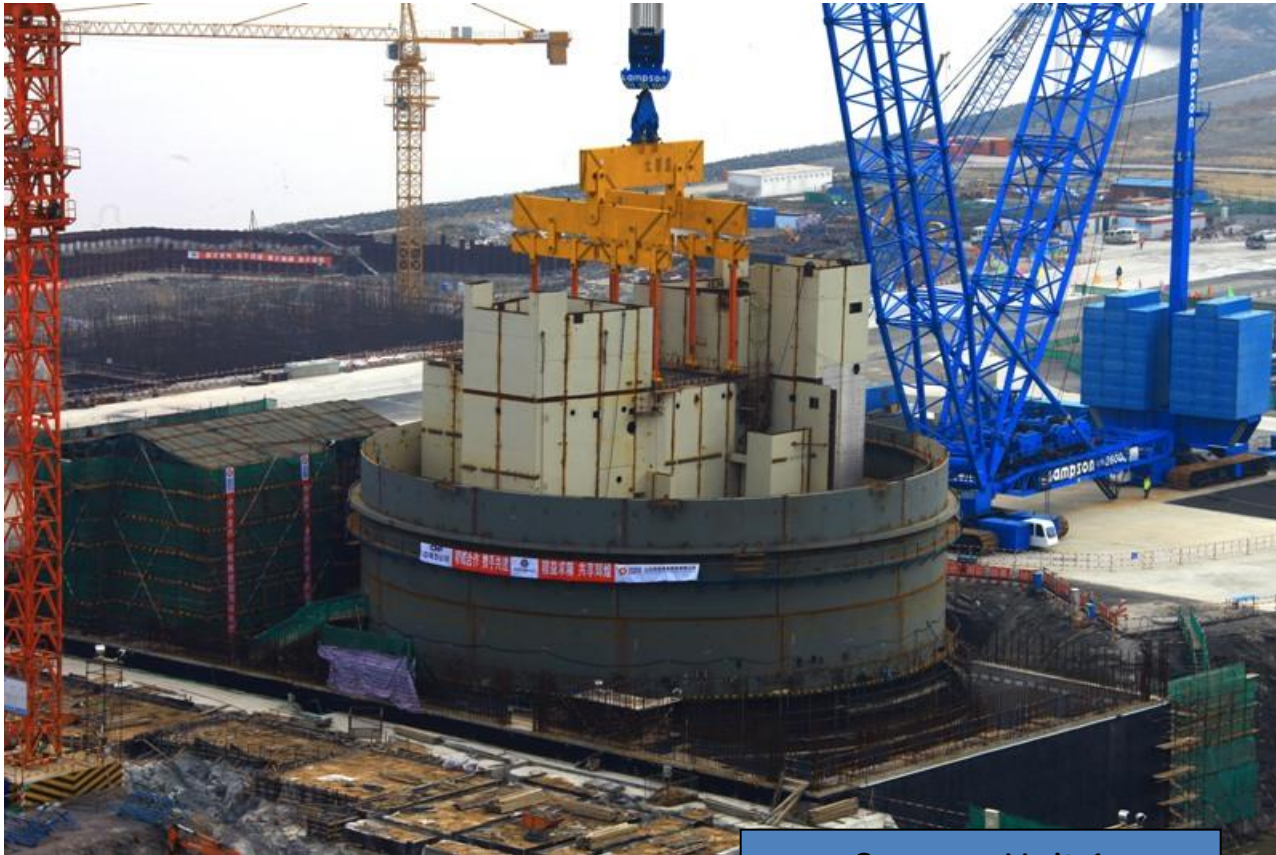
Sanmen Unit 1 March 27, 2010
