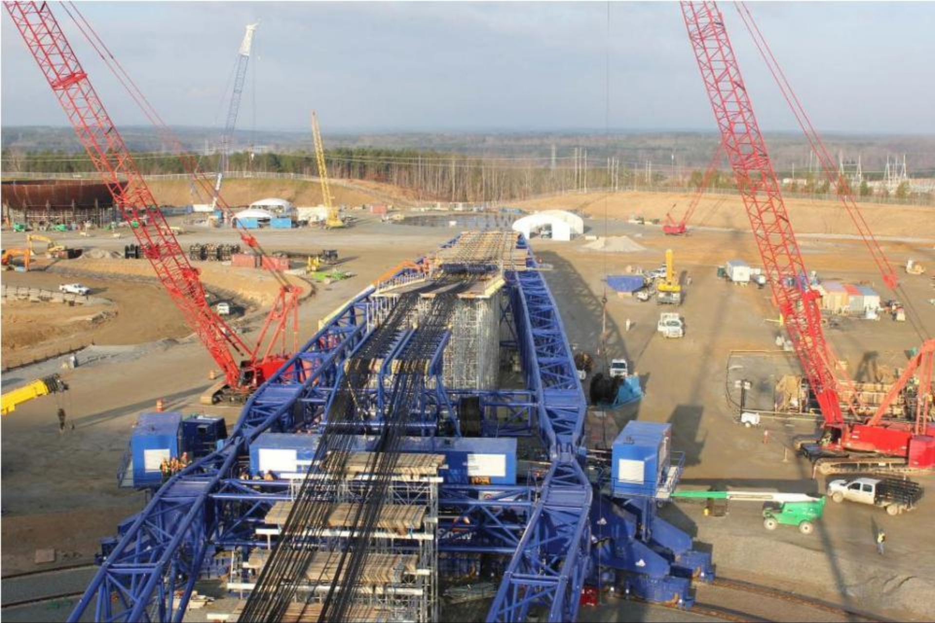
2.22.12 HLD Erection, CBI Vessel Head
